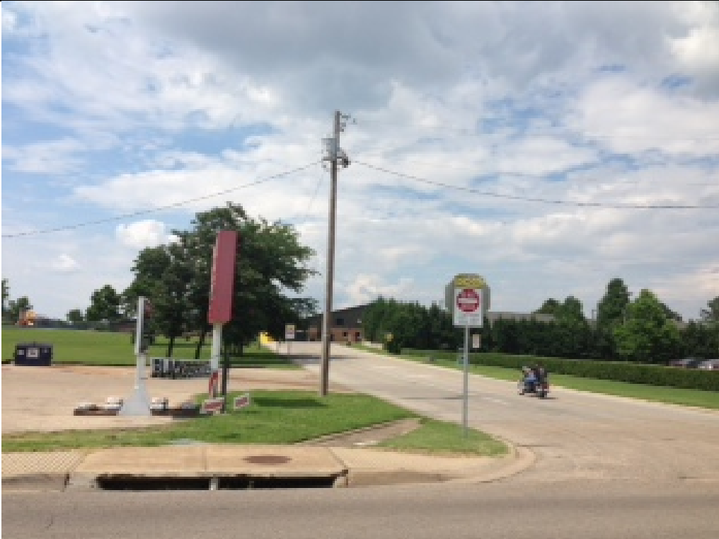
View Looking North at Intersection of Highland & Hillcrest
