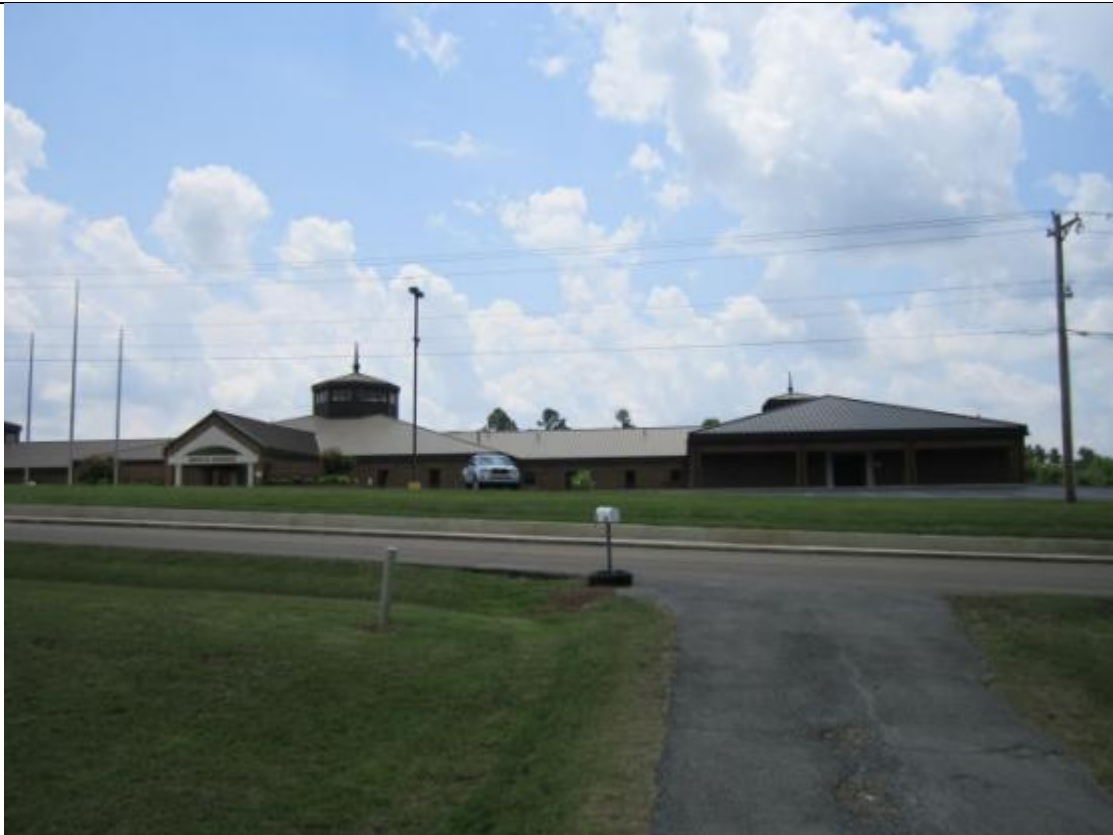
Jonesboro Public Schools Math and Science located southeast of site.
