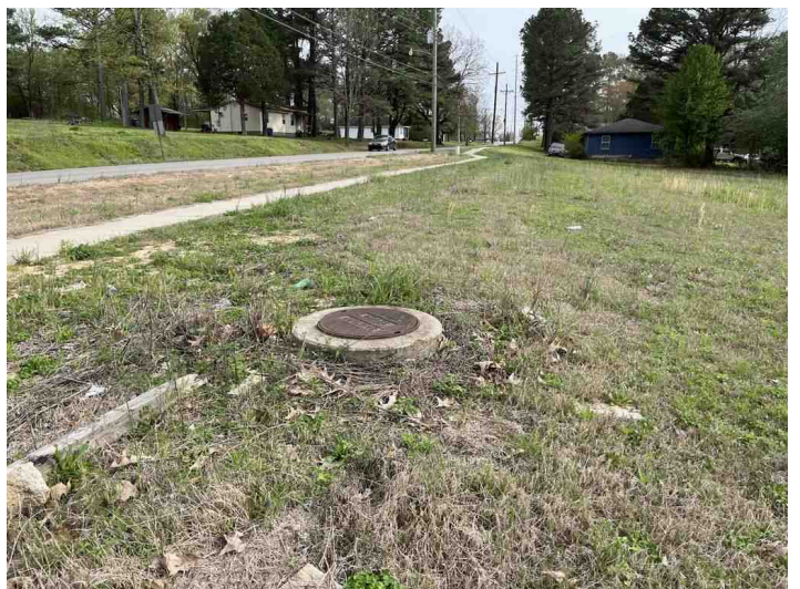
Utilities on Site
