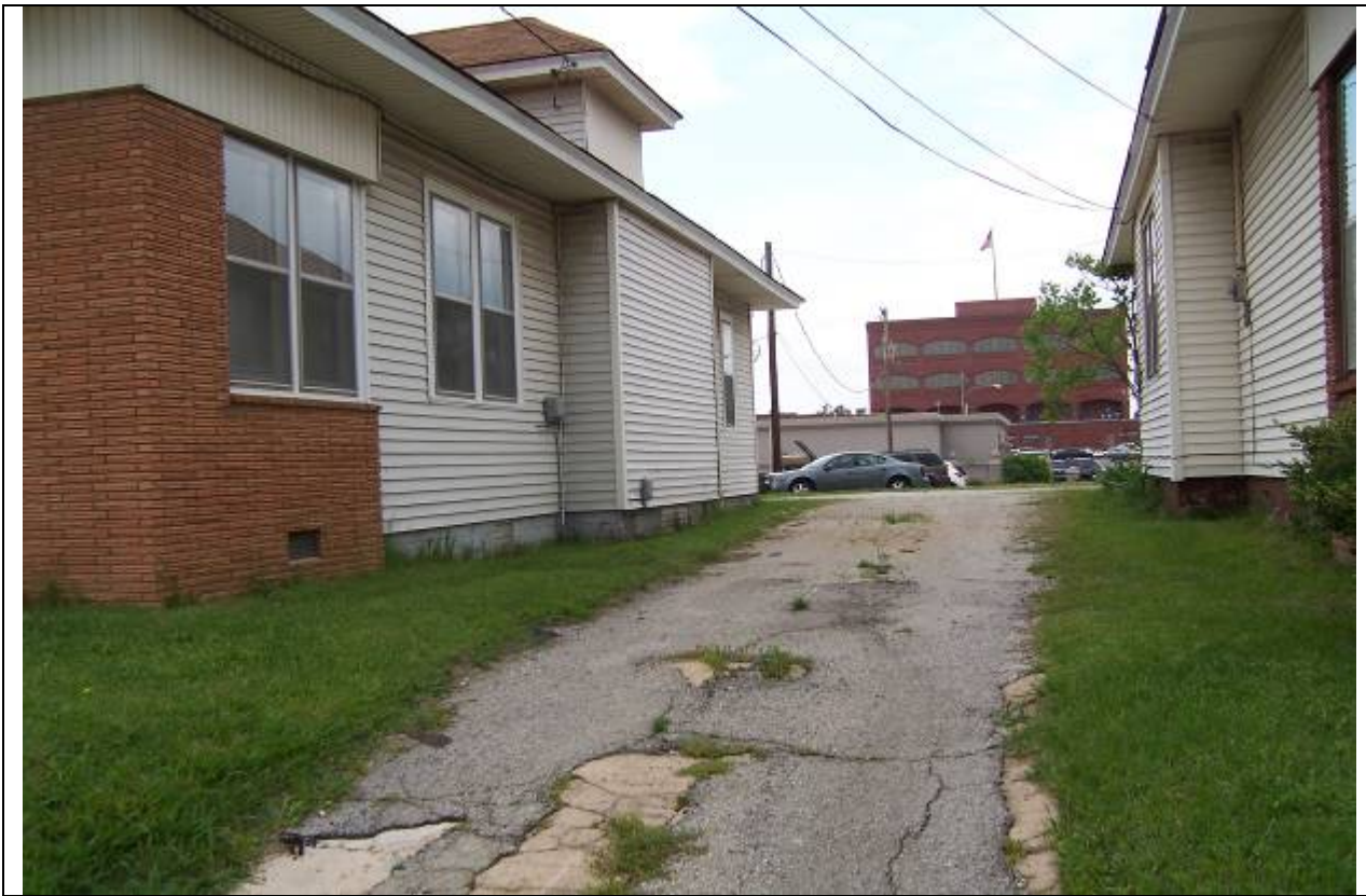
View looking north into rear yard/driveway of project site.
