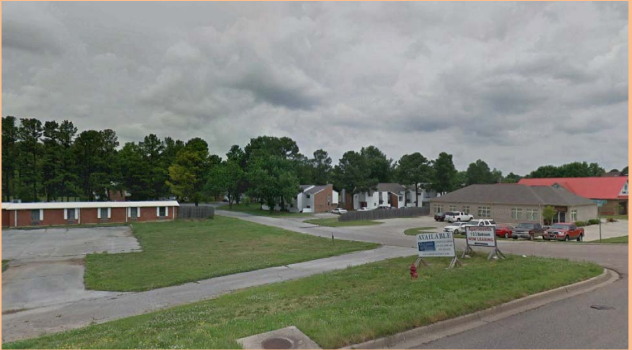
View looking North
