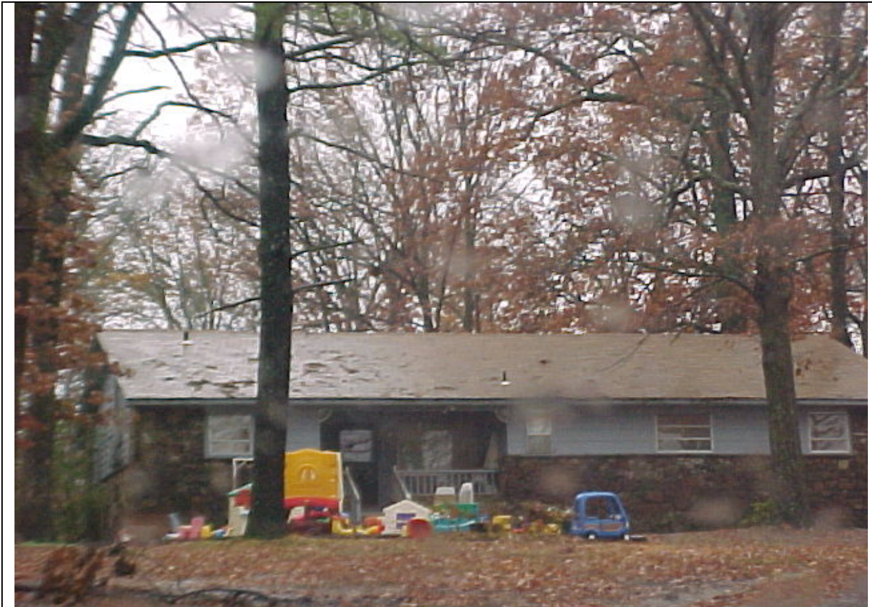
View looking south at the subject site.
