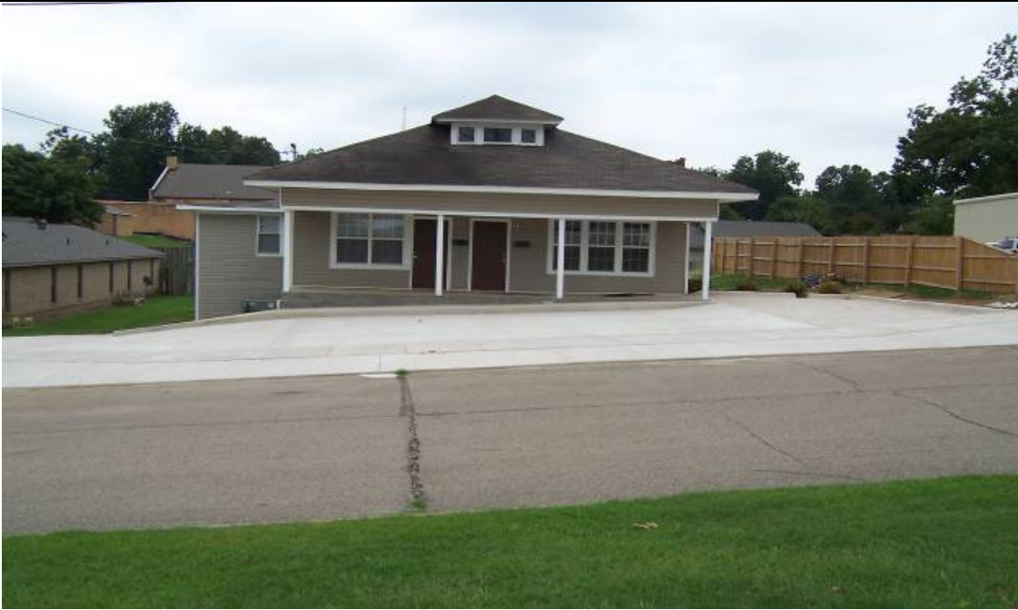
View looking south at property
