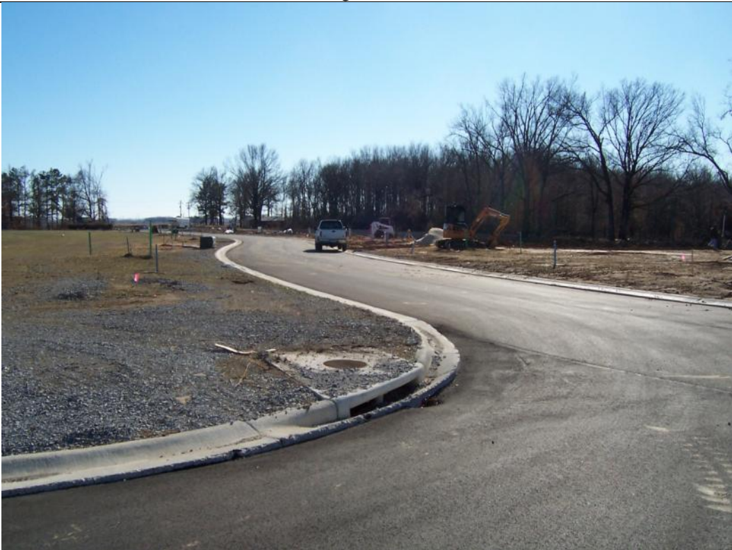
View Looking south
