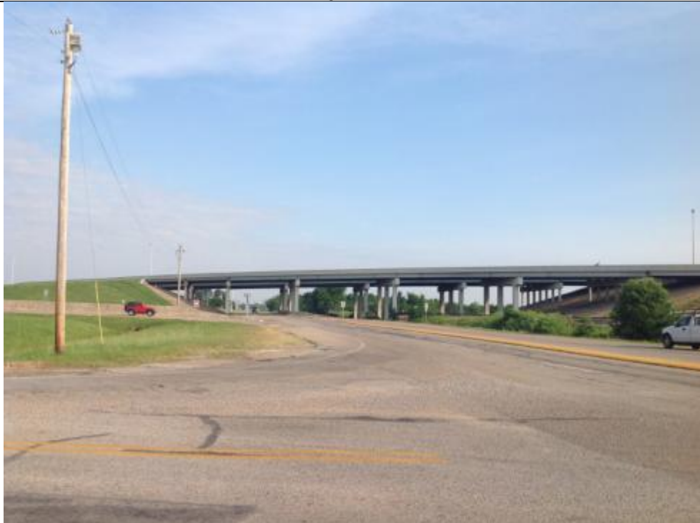
R-1 property located east of site. Jack's Treasures Flea Market, The Treasure Hunt Flea Market, and a body shop to the rear.
