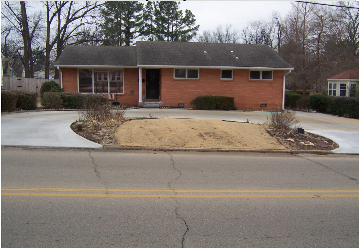
View looking at subject property (principle structure).
