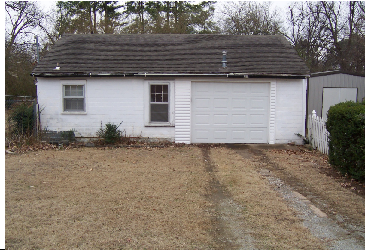
View looking at subject property (accessory dwelling structure) rear yard.
