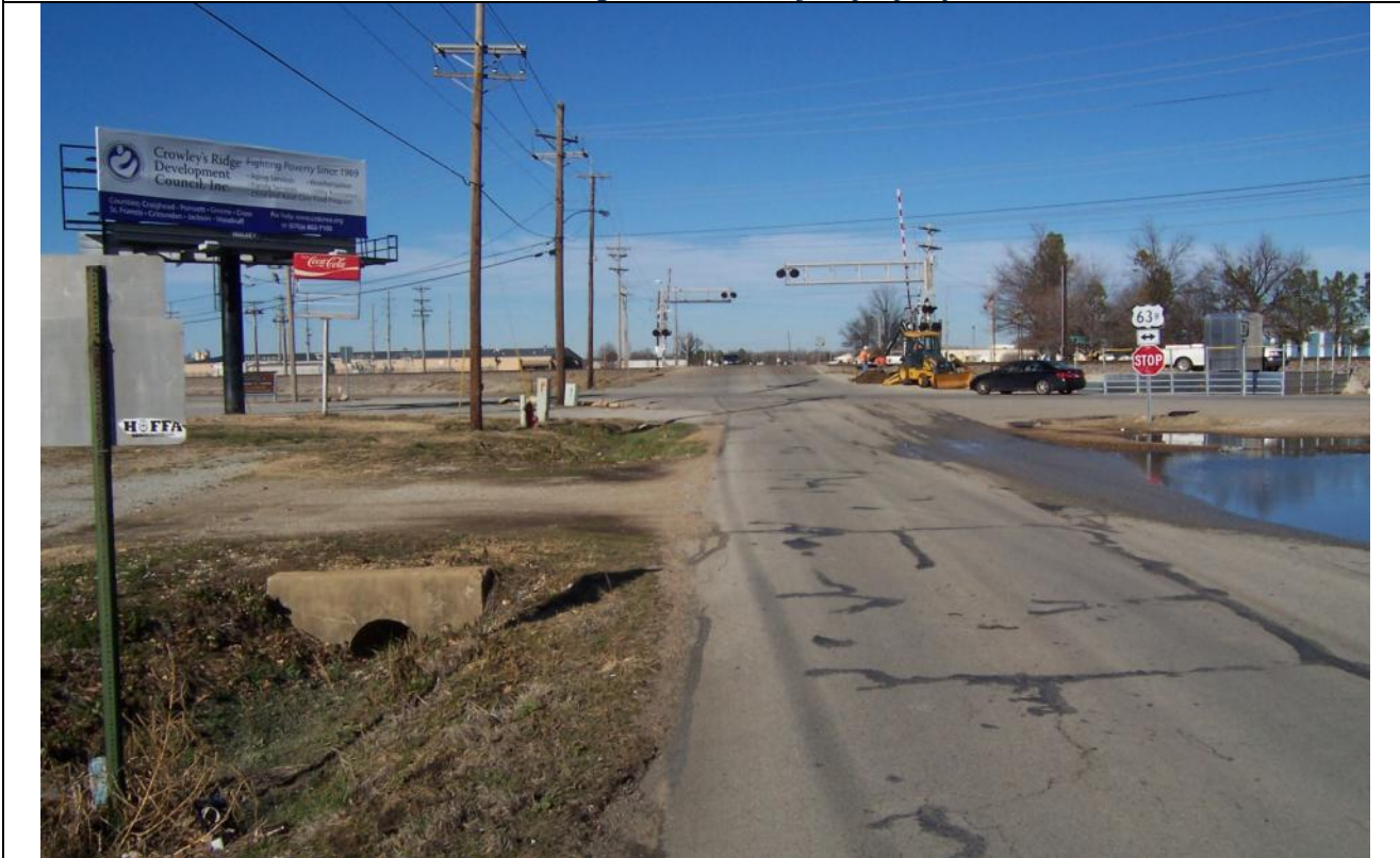
View looking north along Industrial Dr.
