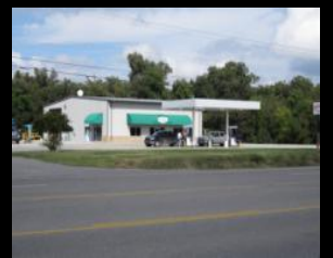
Fig. 5: Example Rural Development Type-Service Commercial-Fueling Station
