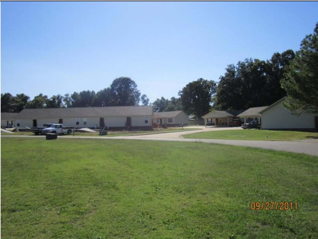
View looking South from the site.
