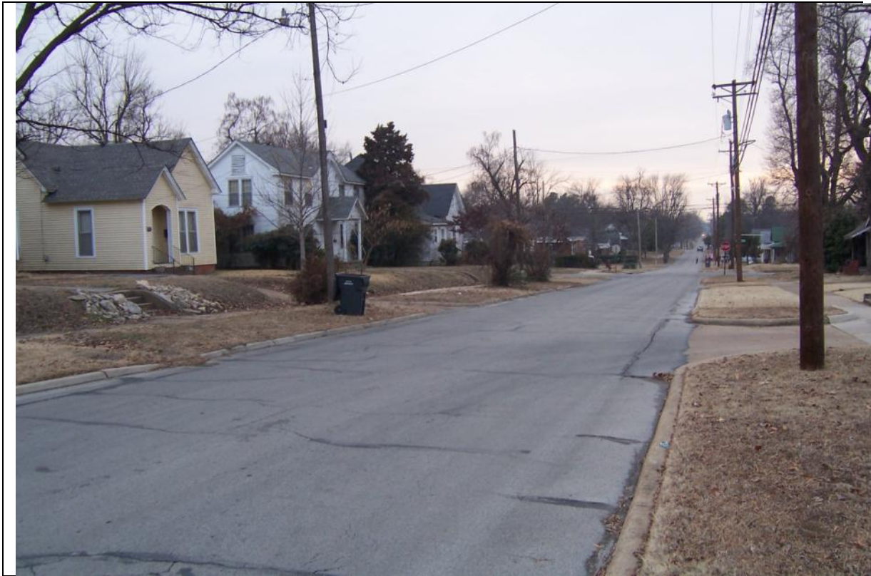
View looking west along Jefferson Ave.
