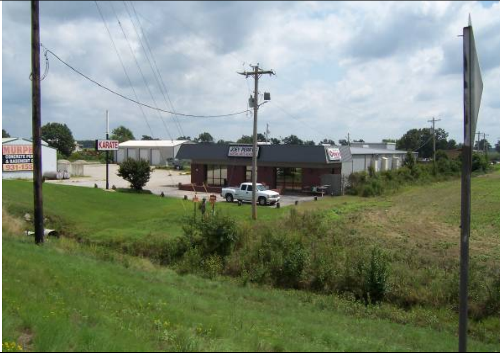
View looking southeast at site
