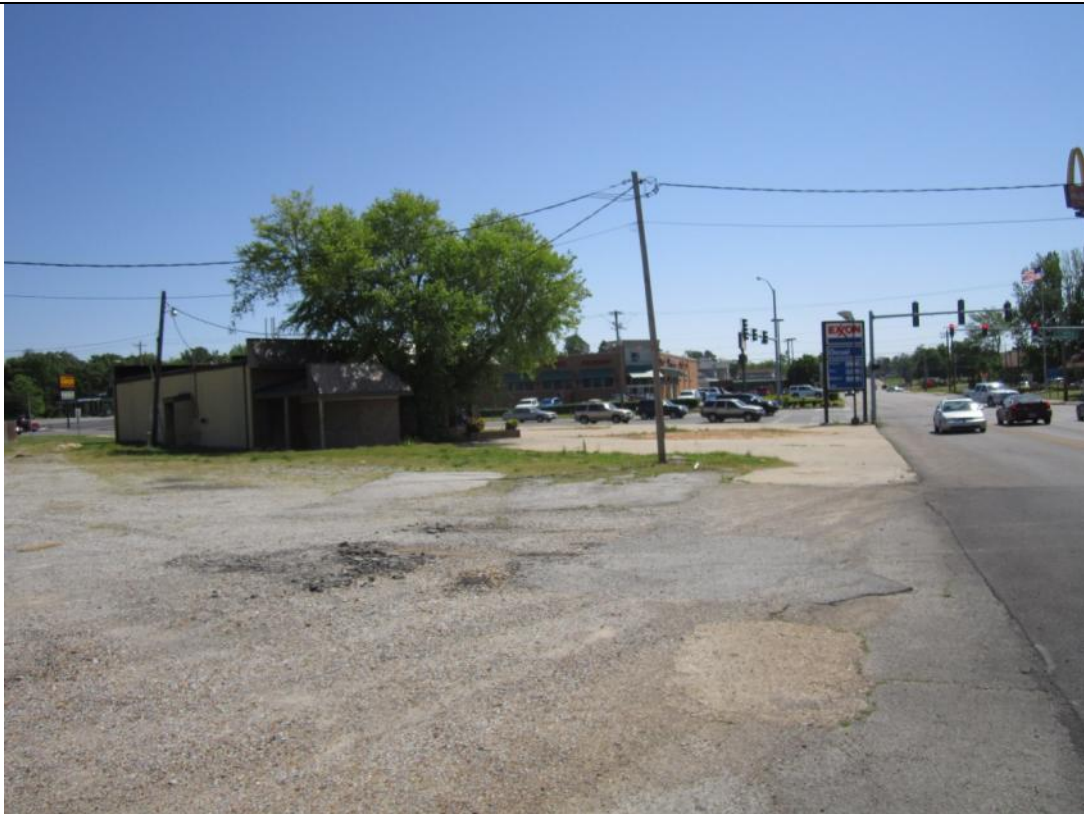
View looking East along Highland Dr. towards existing Exxon Building
