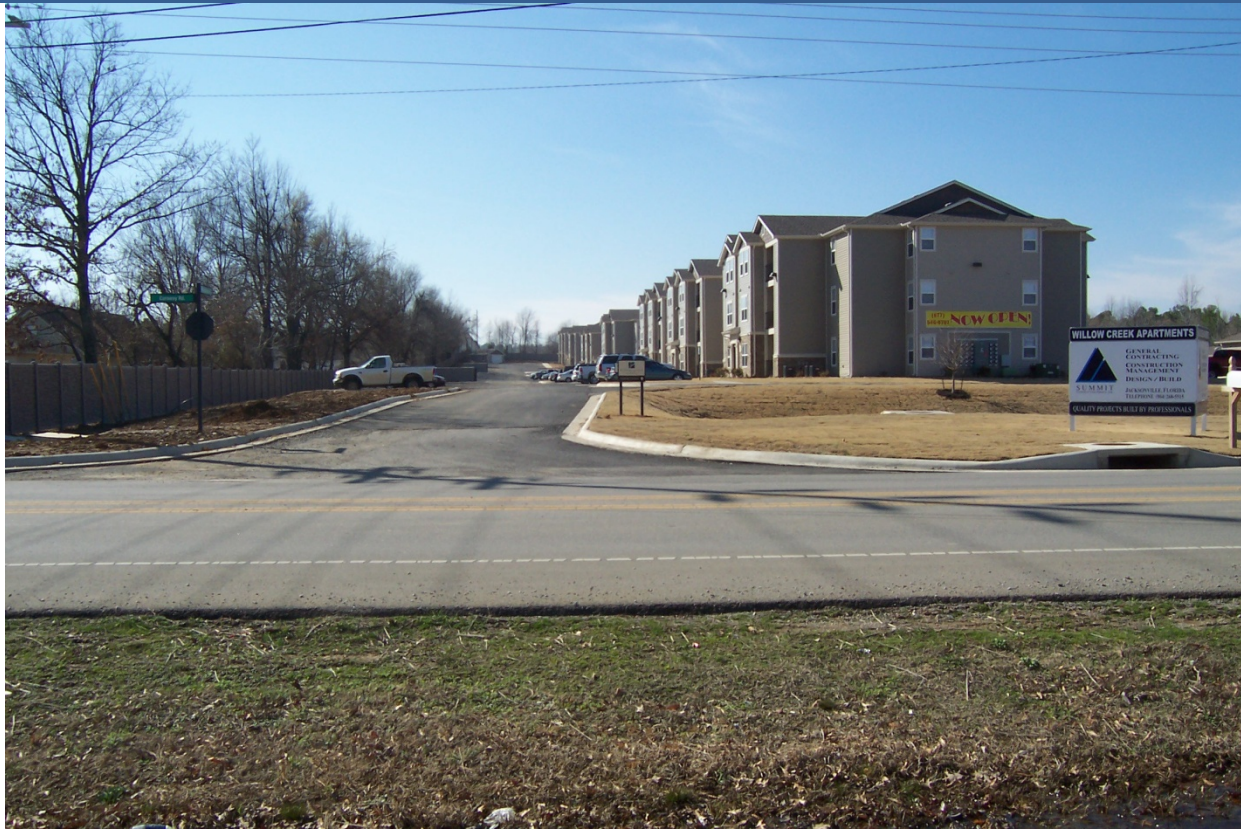
View looking West of apartment entrance (south).
