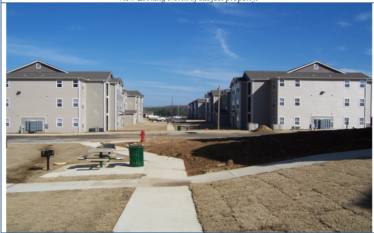
View looking East within the Willow Creek Apartments complex.
