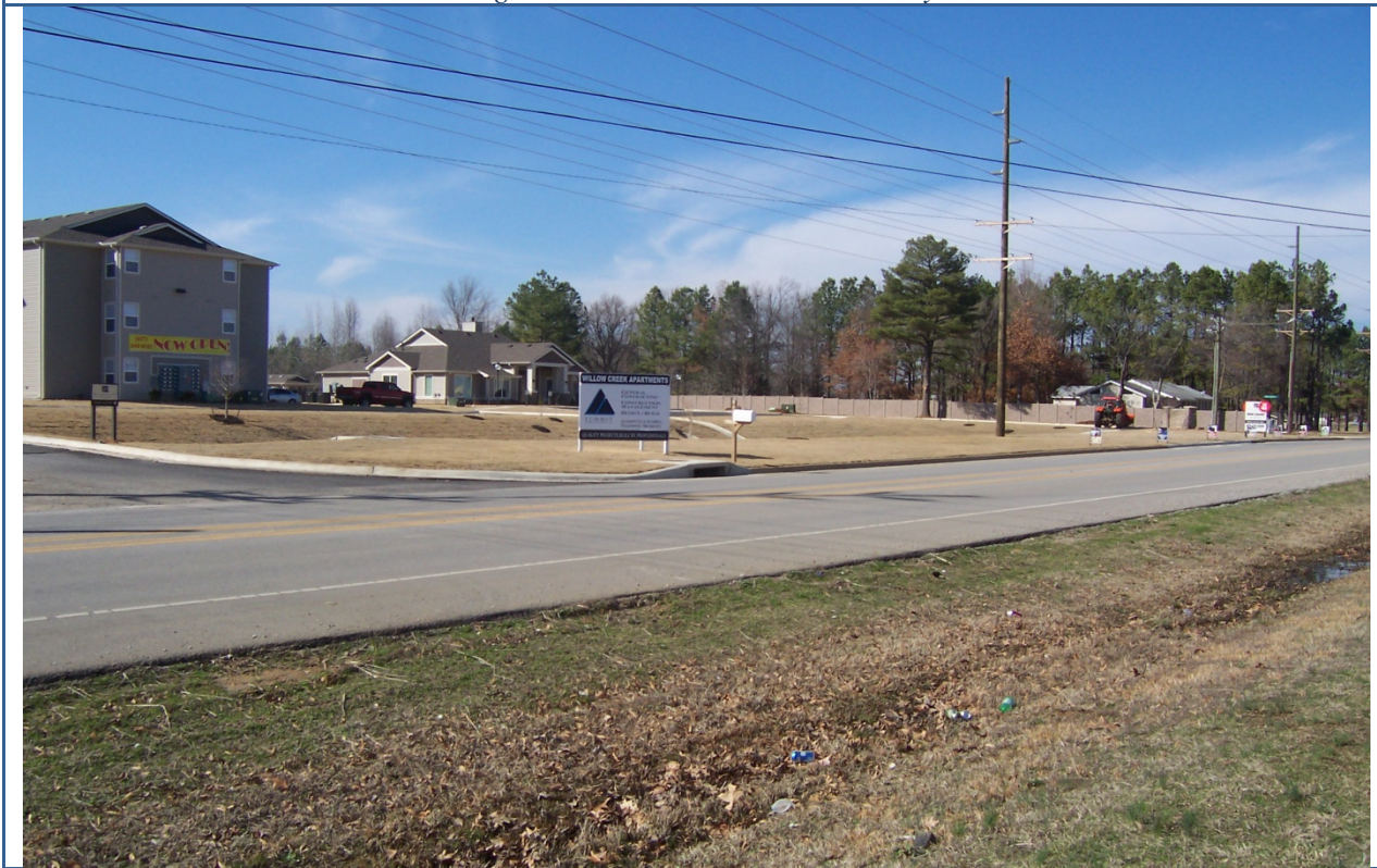
View looking West of Willow Creek Apartments from S. Caraway.
