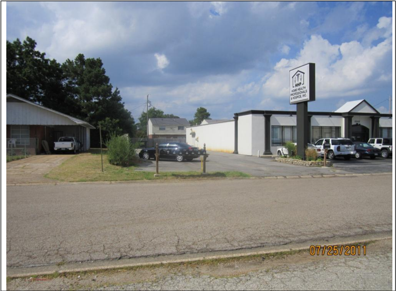
View looking North of abutting commercial property (Home Health Professionals).
