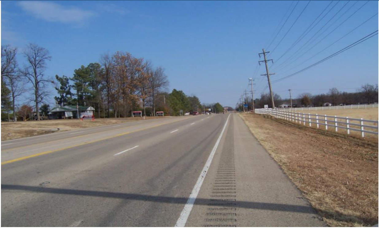
View looking East along Johnson Ave.
