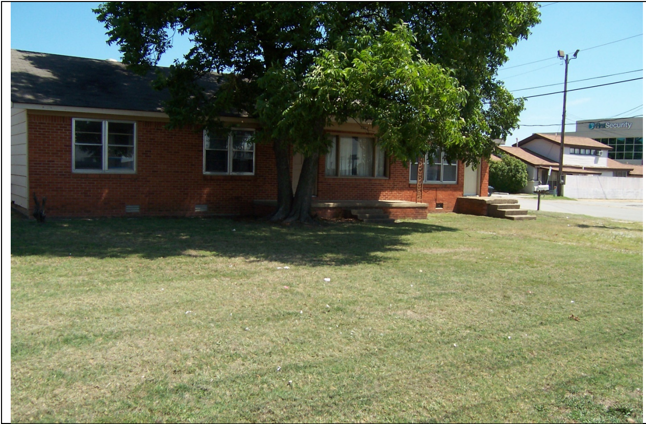
View of existing structure from Nettleton Ave.
