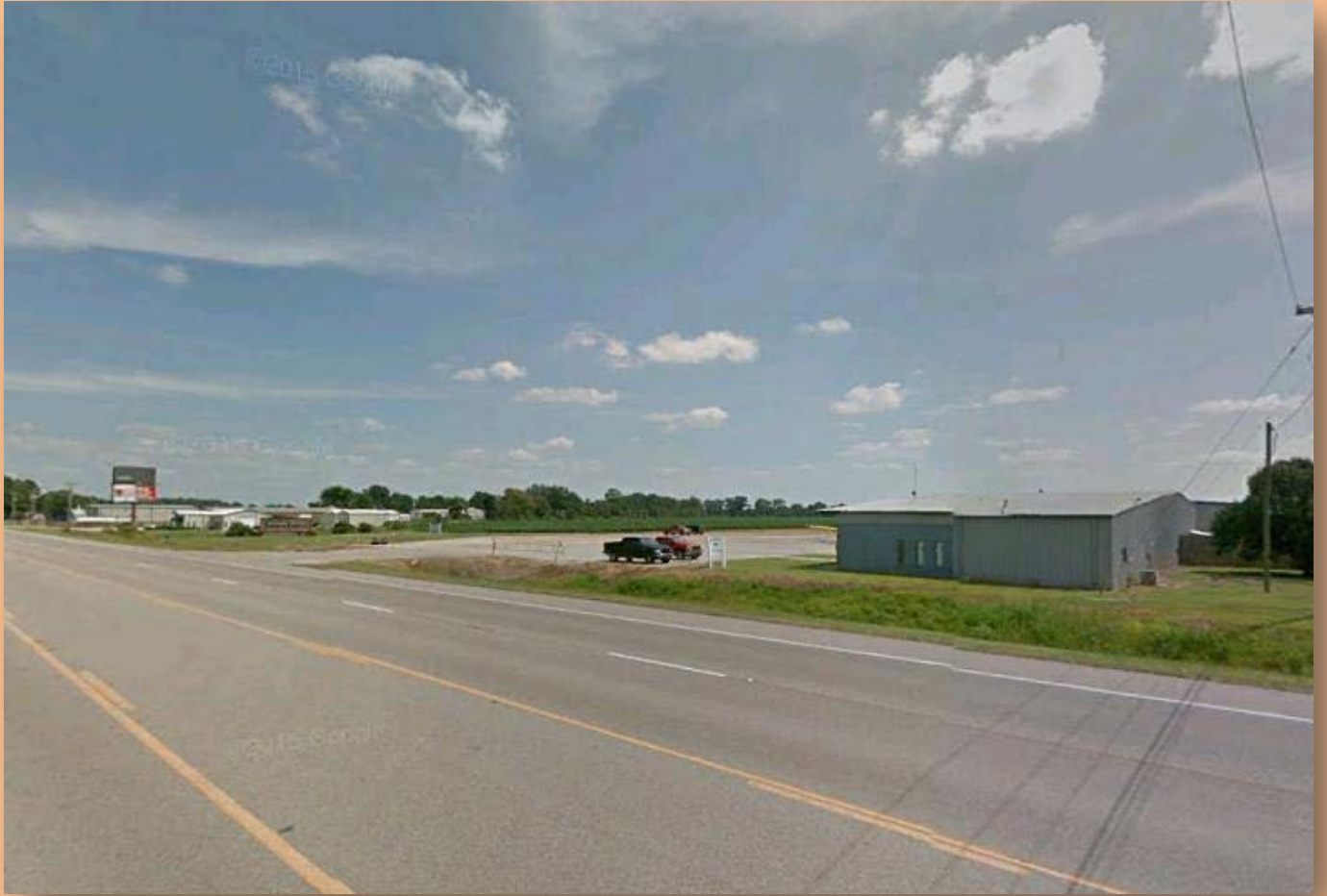
View looking south toward property site
