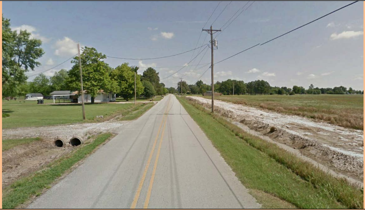
View looking North
