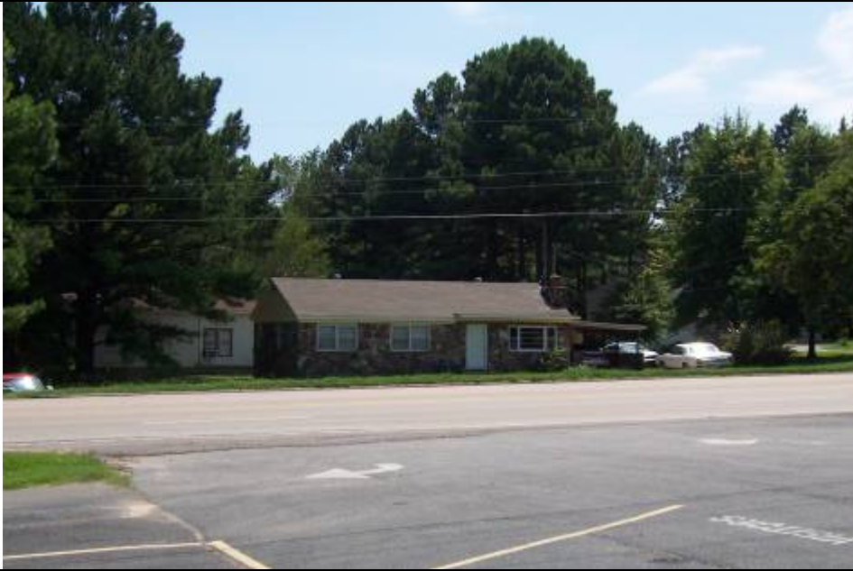
View looking south
