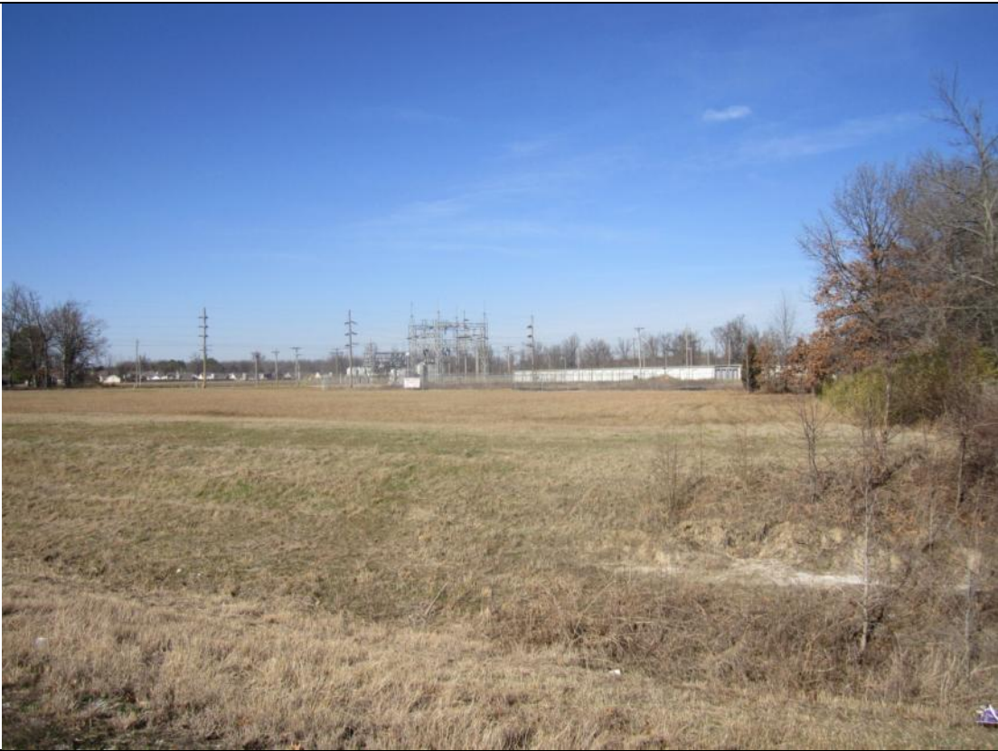
View looking Northwest from Hwy 49 (Farrville Curve).
