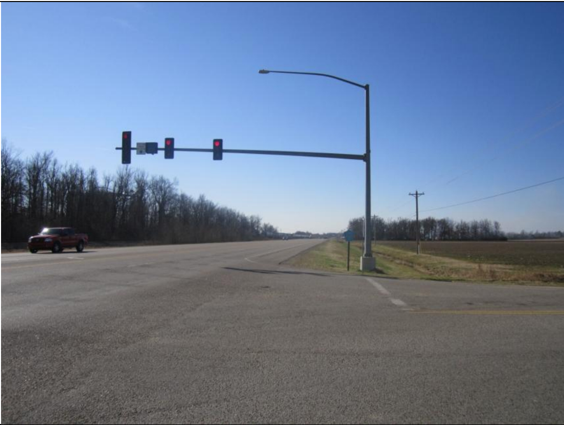
View looking South at Hwy 49/ CR 702 intersection.
