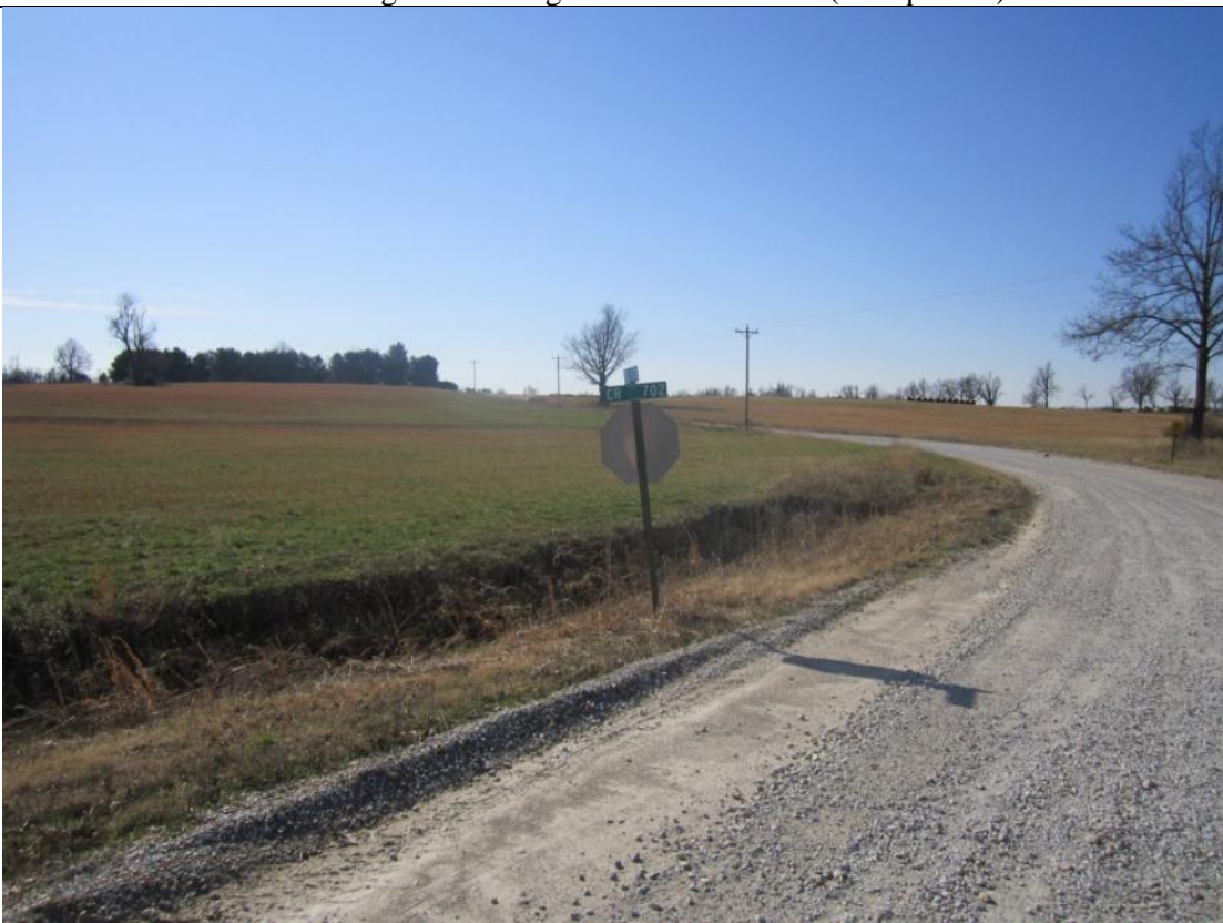
View Looking Southwest along Clinton School Rd./CR 702 (unimproved).
