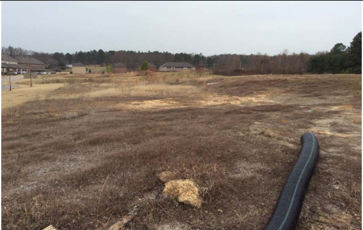
View on Site looking South
