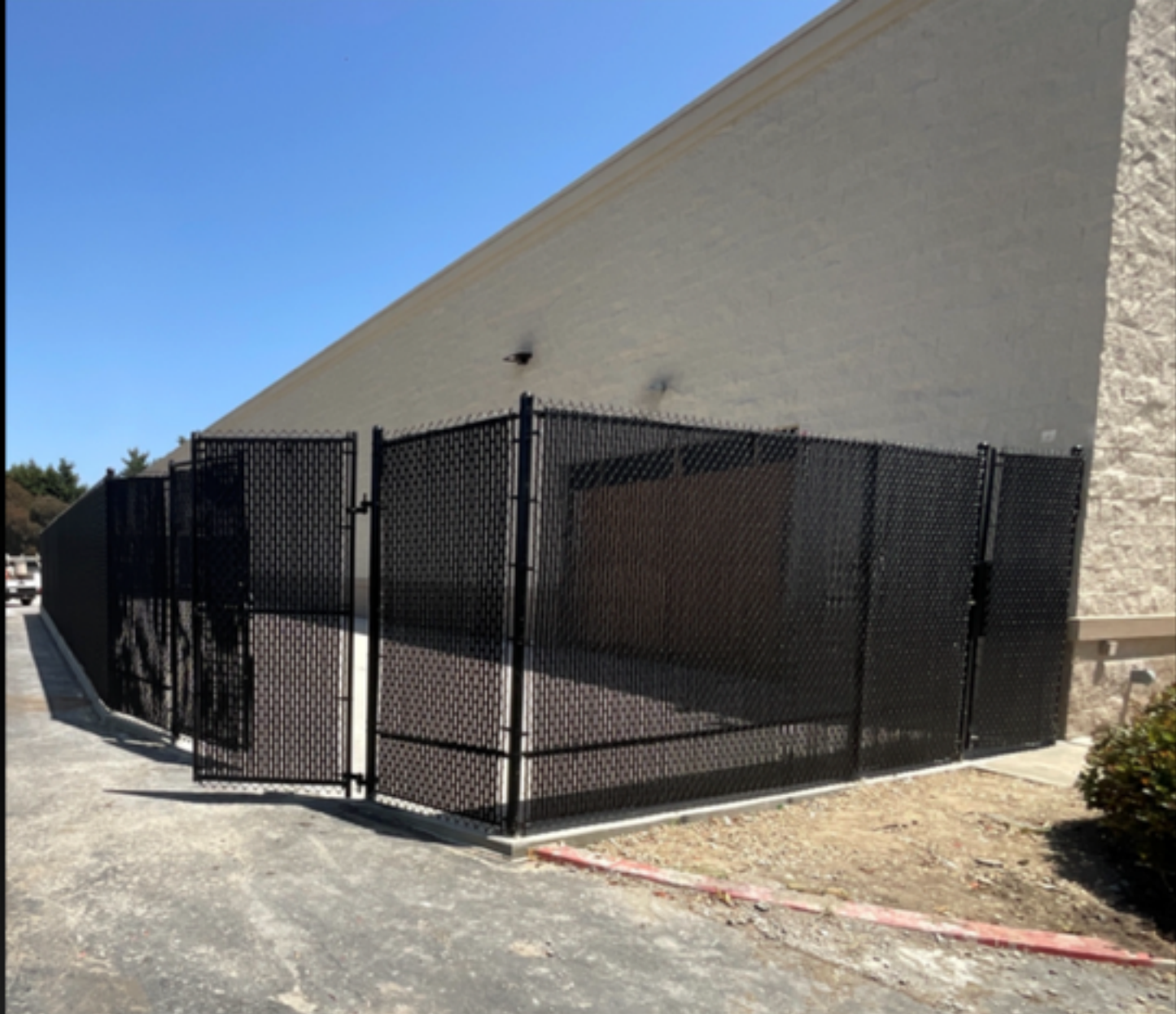
EXAMPLE BLACK CHAINLINK FENCE WITH FABRIC SCREEN
