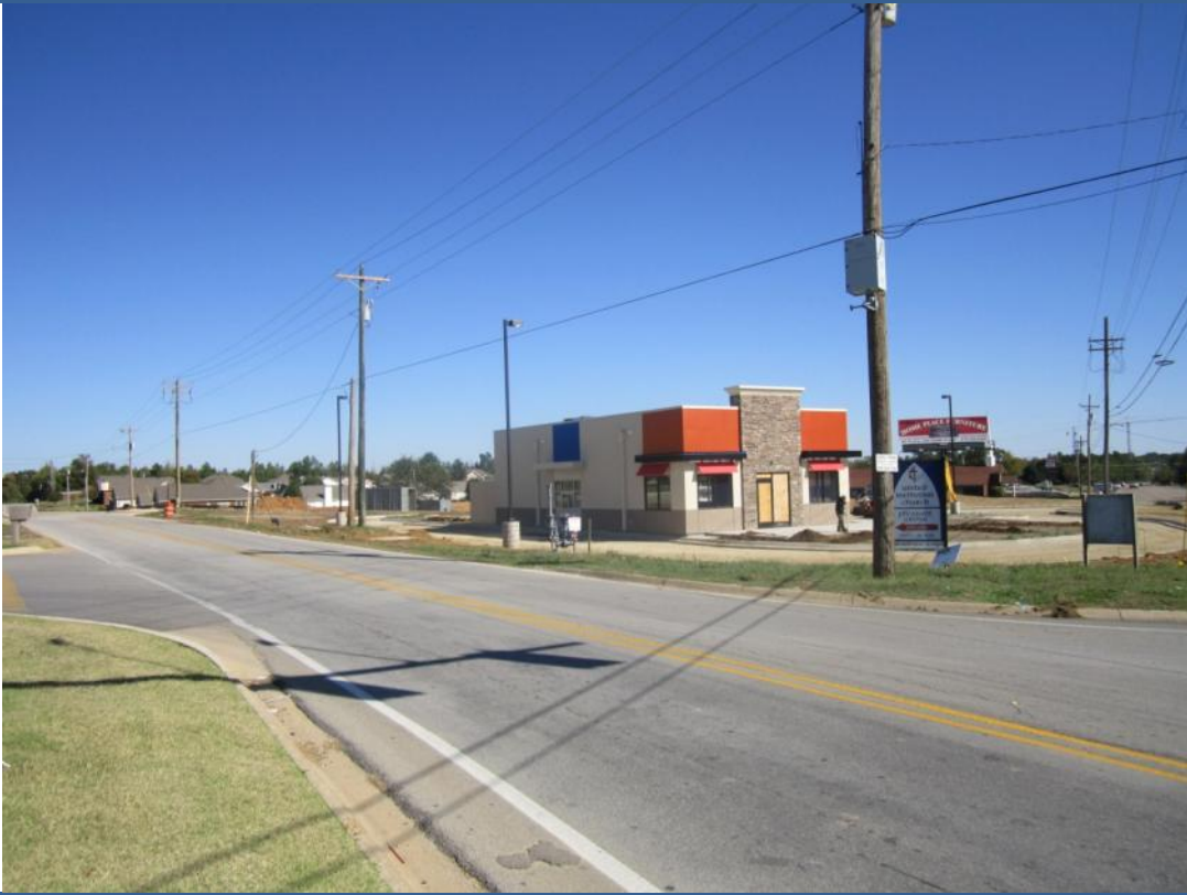
View looking North along Pleasant Grove Rd.
