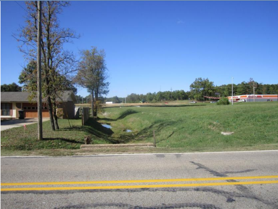
View looking West of subject property (drainage ditch abutting).
