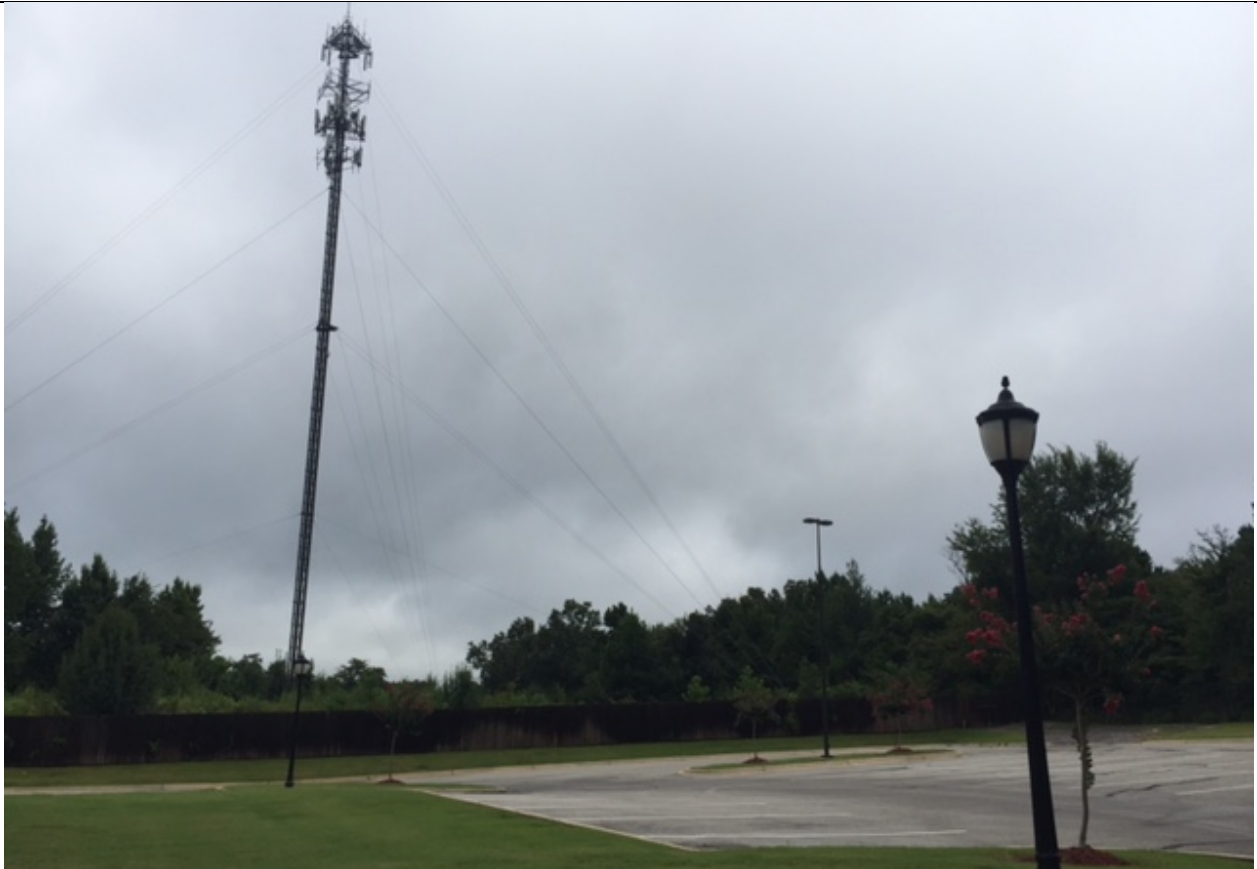
View looking from Wolf Creek Student Apts., North entrance of subject property
