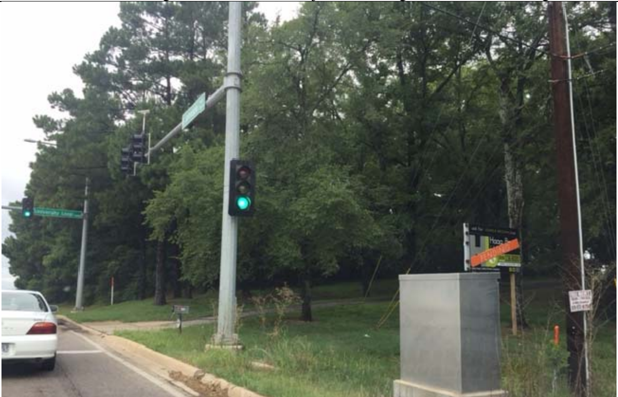
View looking West towards Entry of the Subject Site Along Johnson Ave. Frontage
