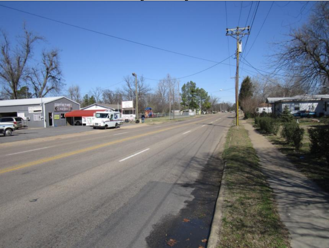
View looking North along N. Main St.
