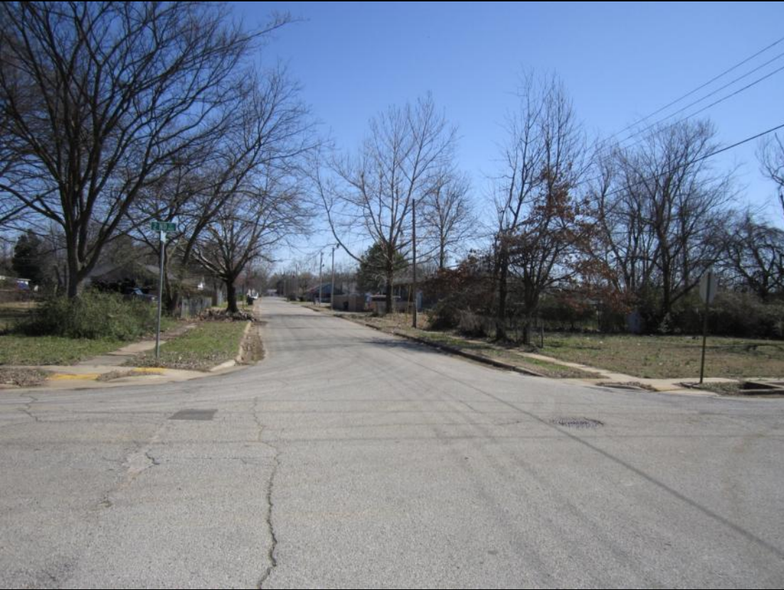
View looking East along Gordon St.
