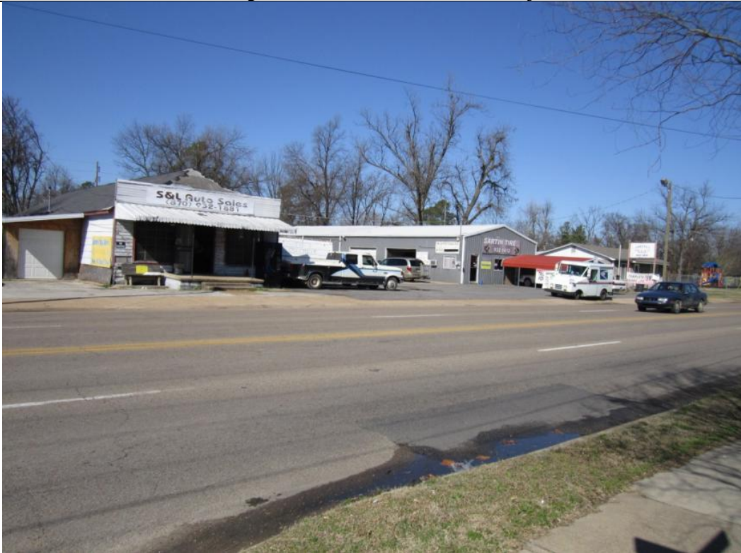
View looking Northwest of Applicant's existing Tire Service along N. Main St.
