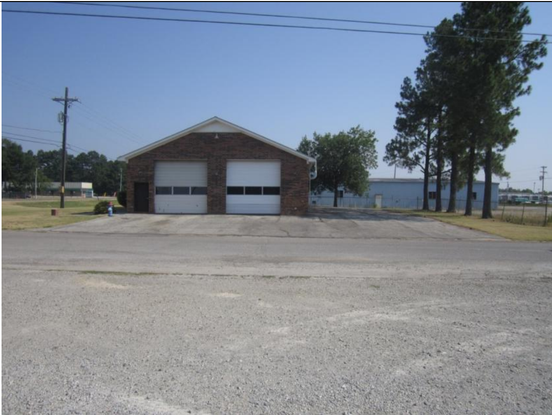
View looking North from adjacent property.
