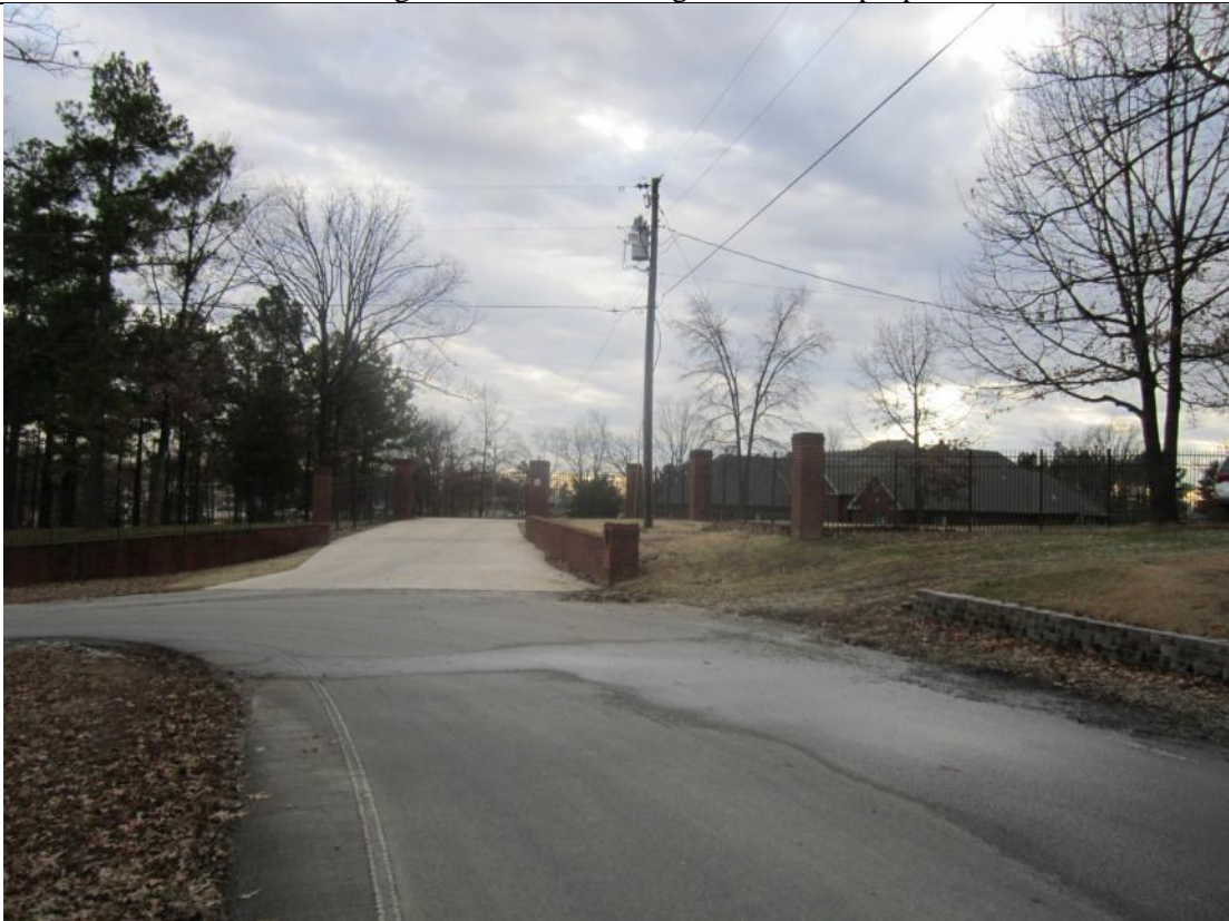
View looking south of the subject property.
