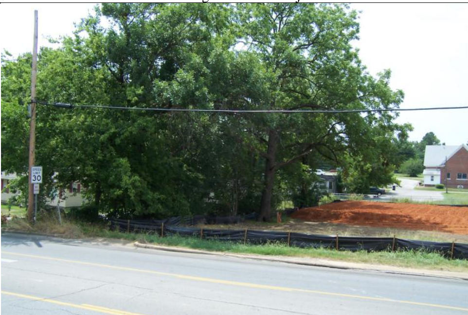
View of the site looking South
