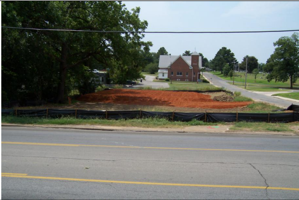
View of the site looking South
