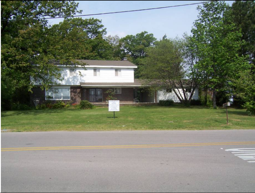
View looking west at subject site
