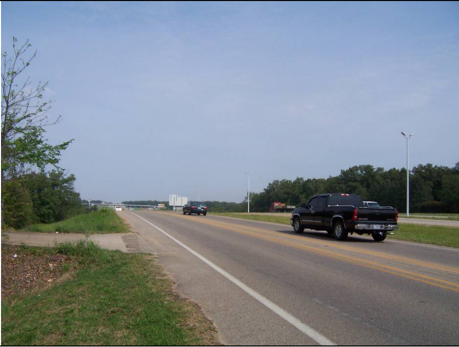
View looking westerly along Parker Rd.
