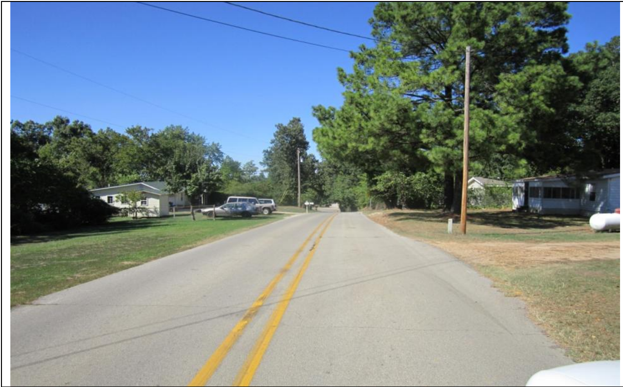
View looking north of abutting residences.
