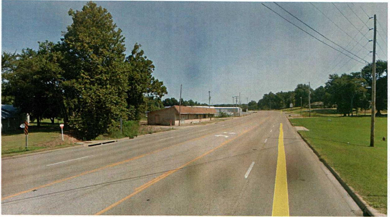
View looking North
