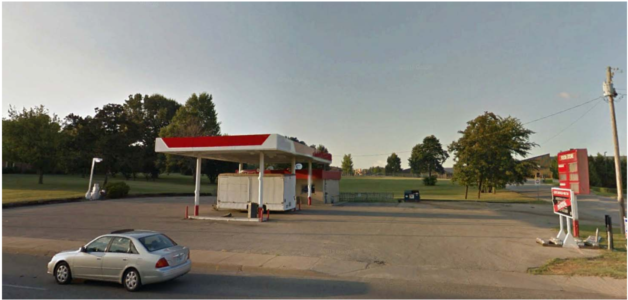
View looking North at Site
