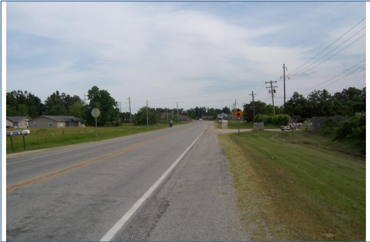
View looking South towards Harrisburg Rd.
