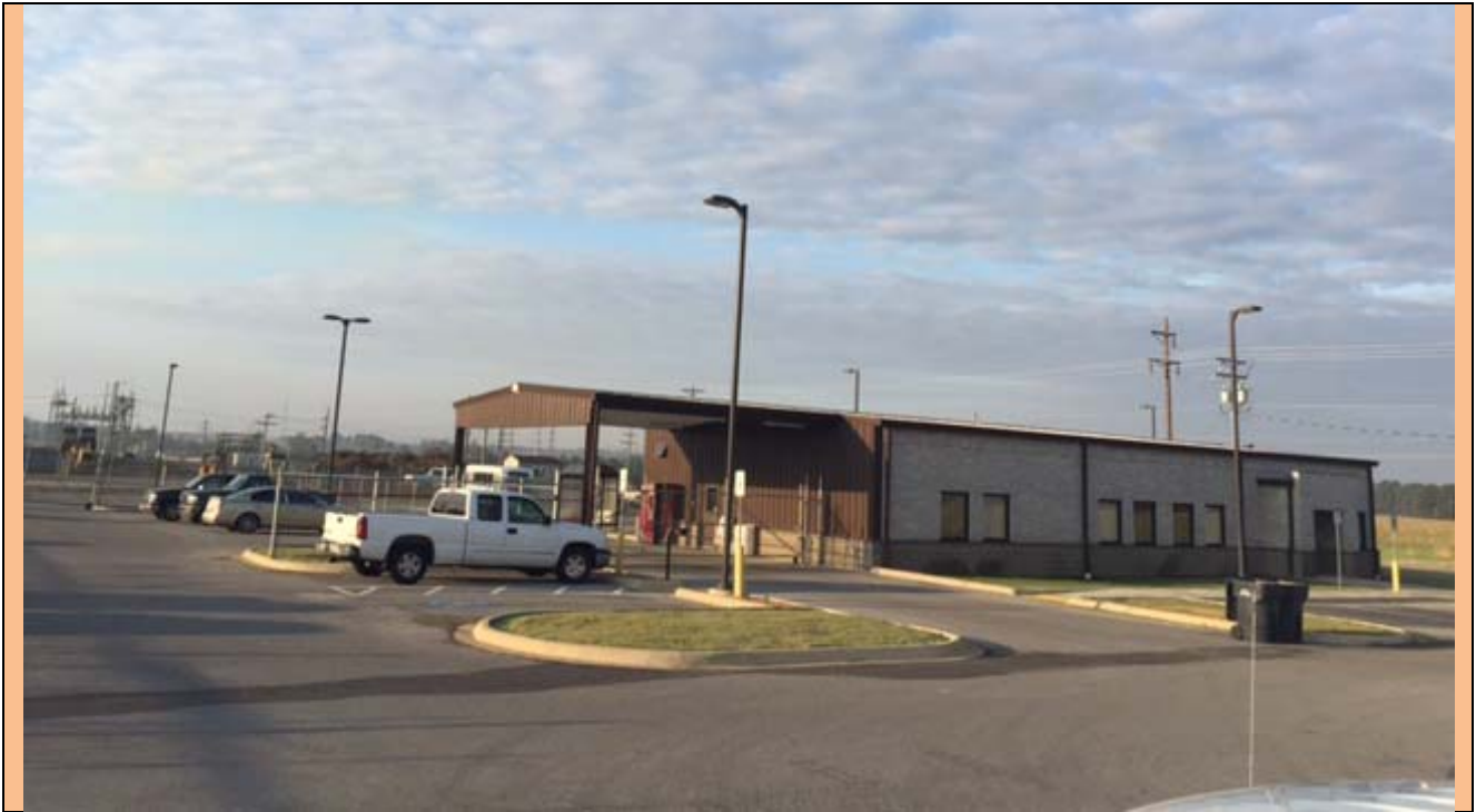
View looking South Towards Jets Facility
