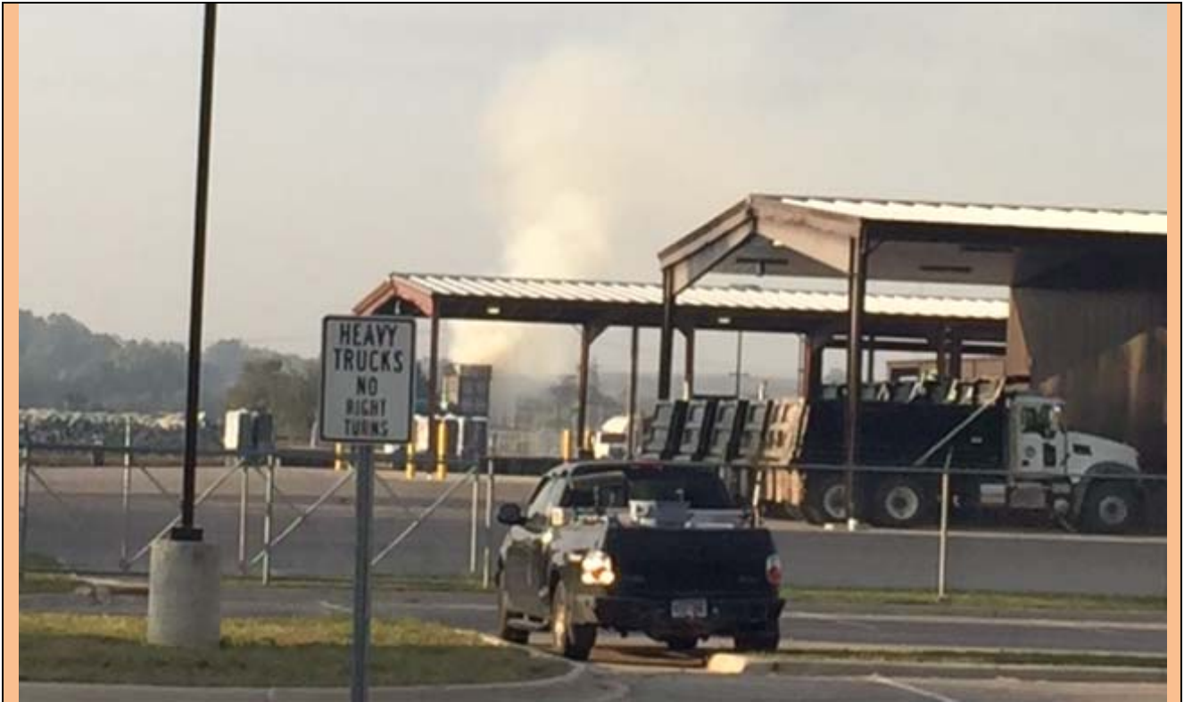
View Looking South on Public Works Facility Property
