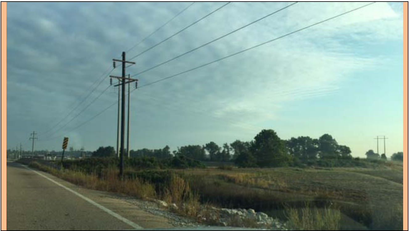
View looking Northeast on Lacy Road South of Public Works Facility
