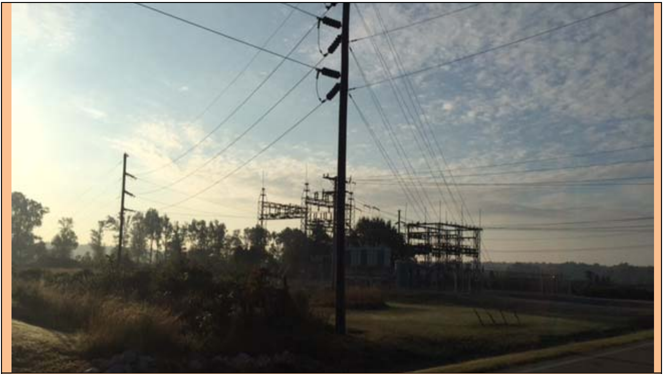
View looking North on Current Public Works Facility Location
