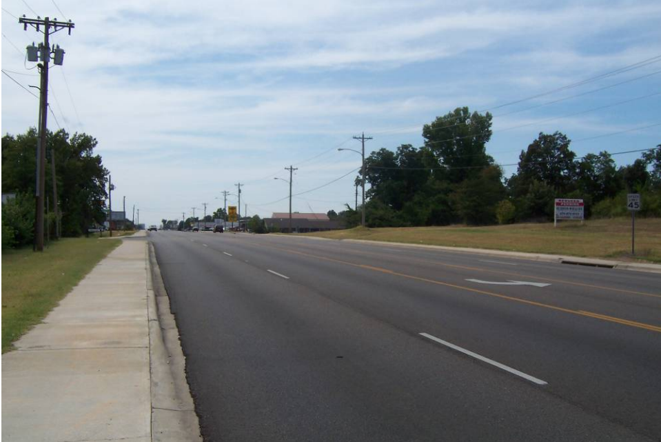
View looking Northeast along Johnson Ave.
