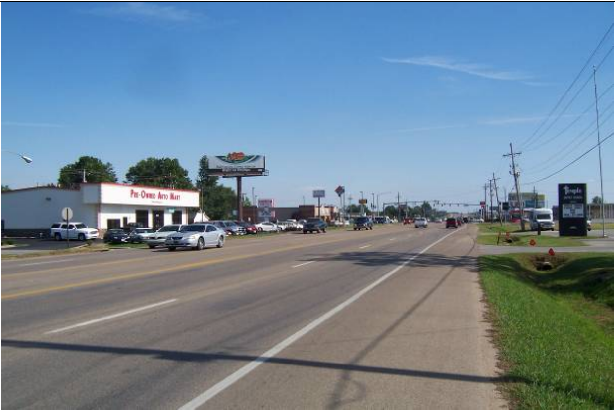
View looking South on Stadium Dr.
