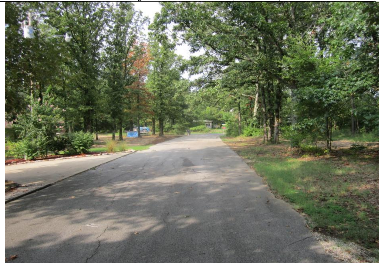
View looking south along Jonkers Circle.
