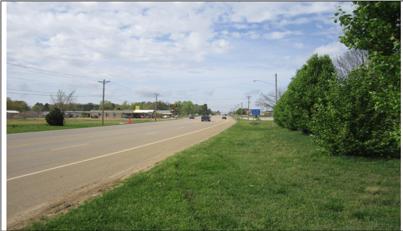
View looking easterly along Highway 49N
