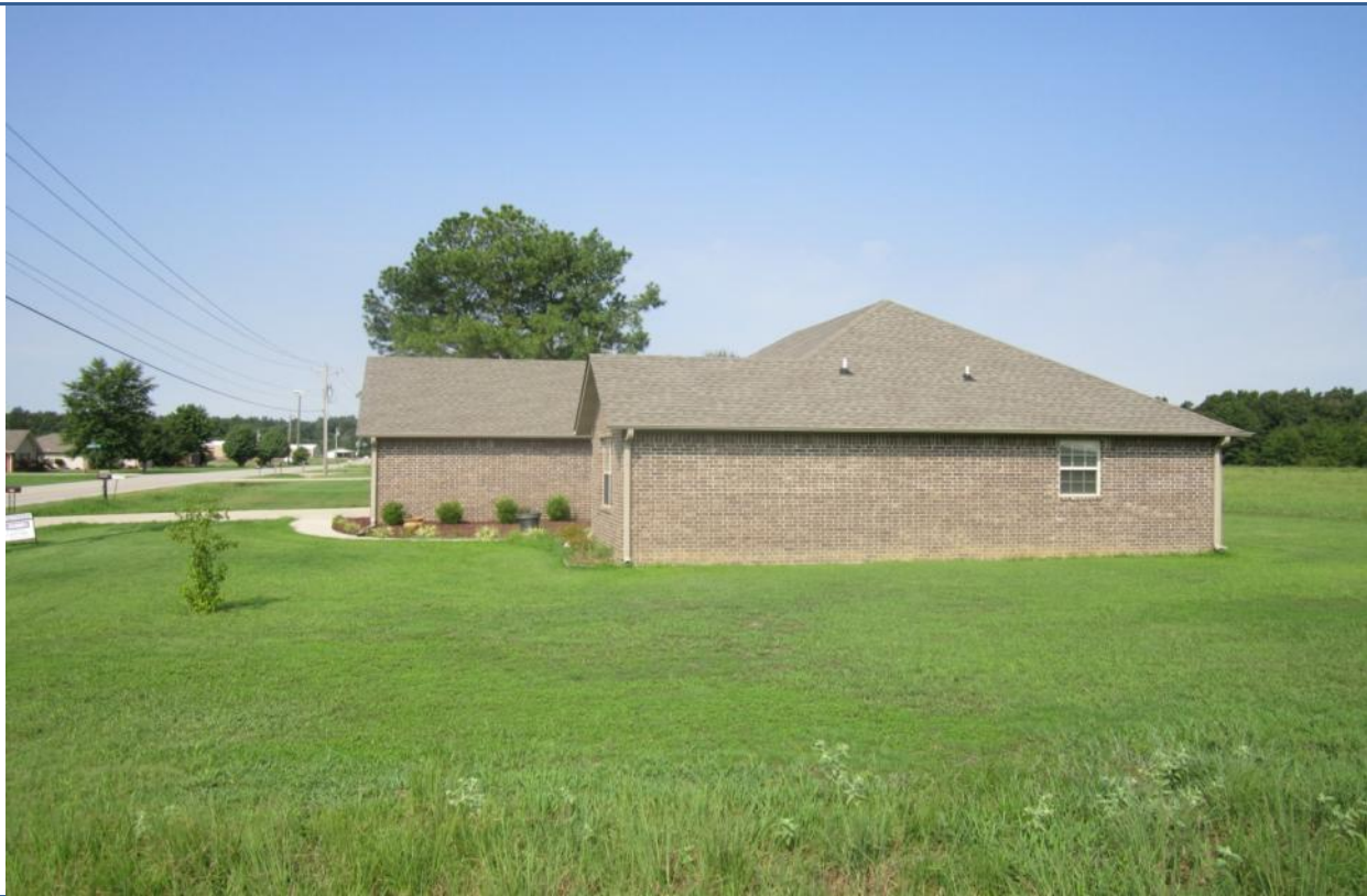
View looking West of home abutting subject property.
