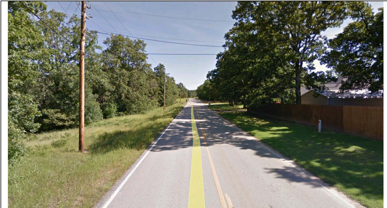
View looking north on Friendly Hope Rd.
