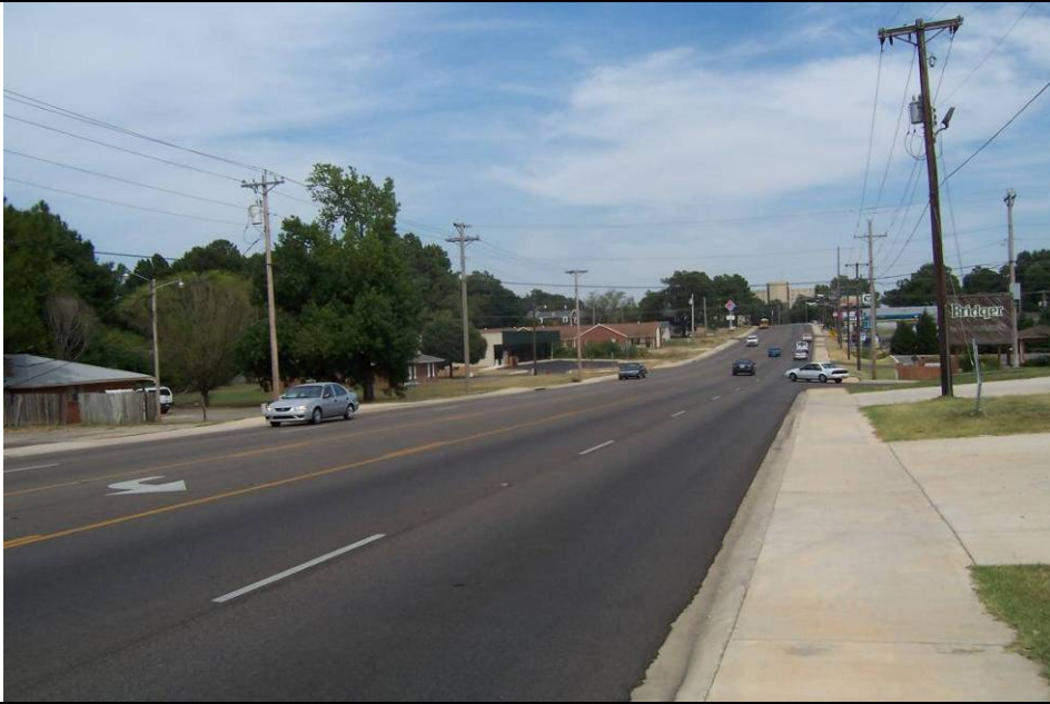
View looking Easterly along Johnson Ave.
