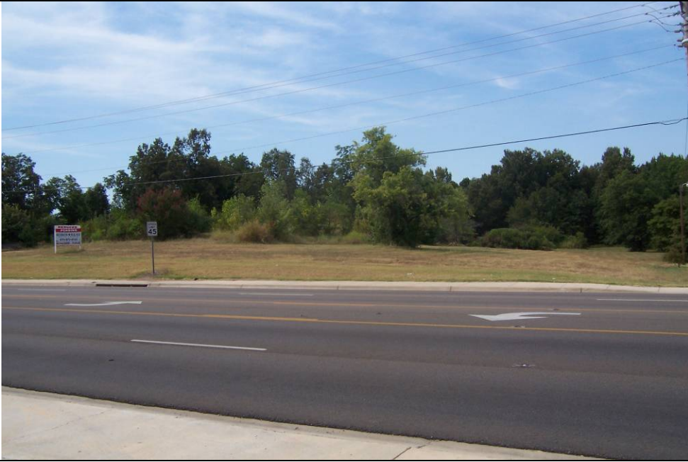
View looking North Along Johnson Ave.
