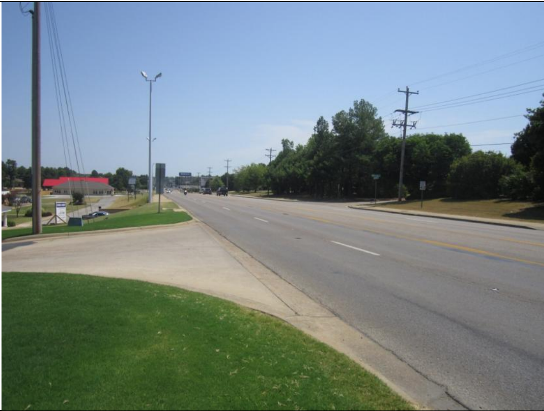
View looking Northeast along Southwest Dr.
