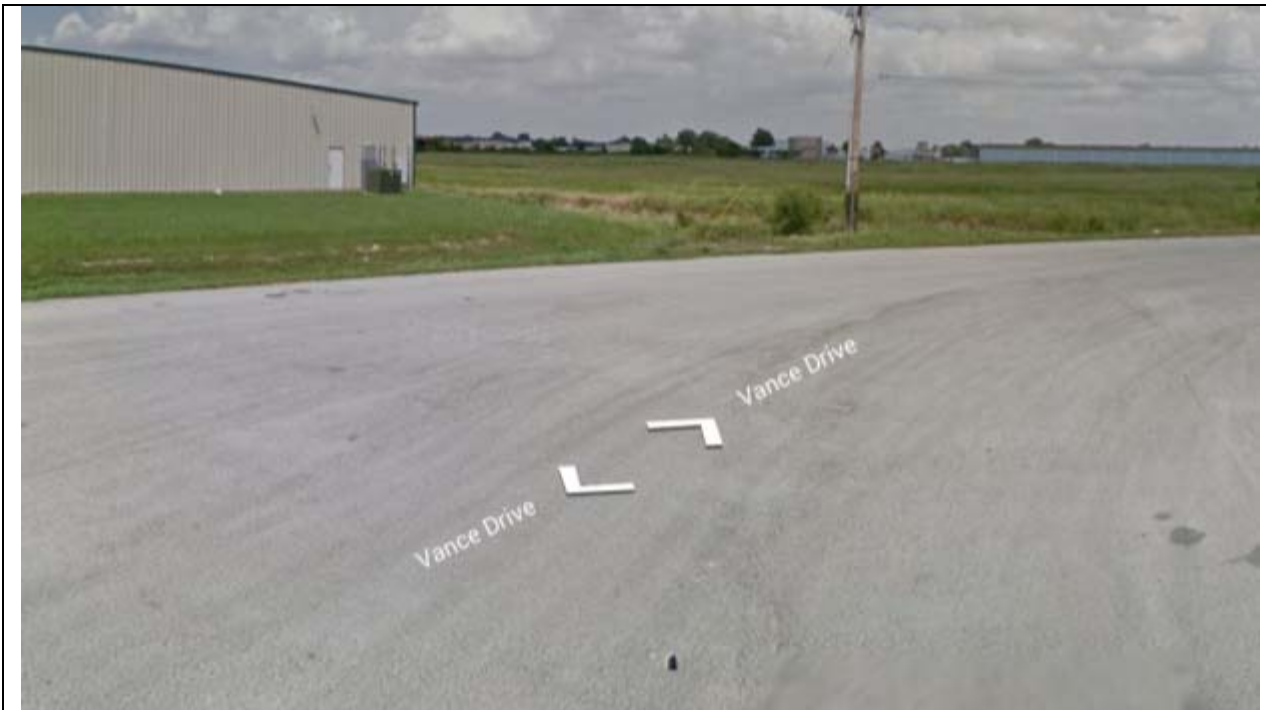
View looking Northeast along toward the terminus of Vance Drive
