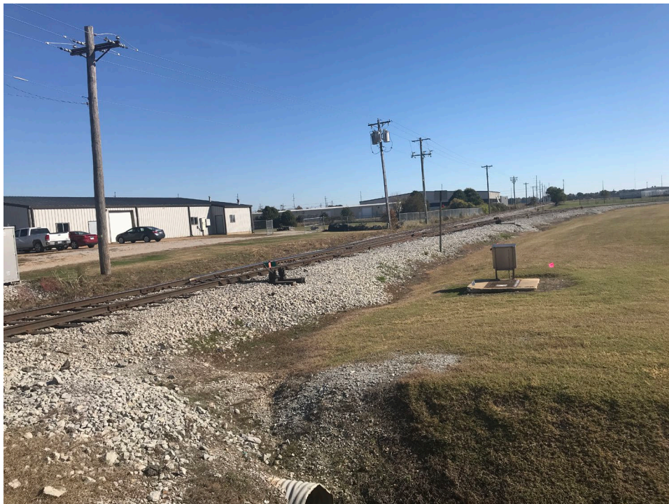
DESCRIPTION: Acquisition Left facing INITIALS: JLA DIRECTION: E DATE: 11/5/2020
