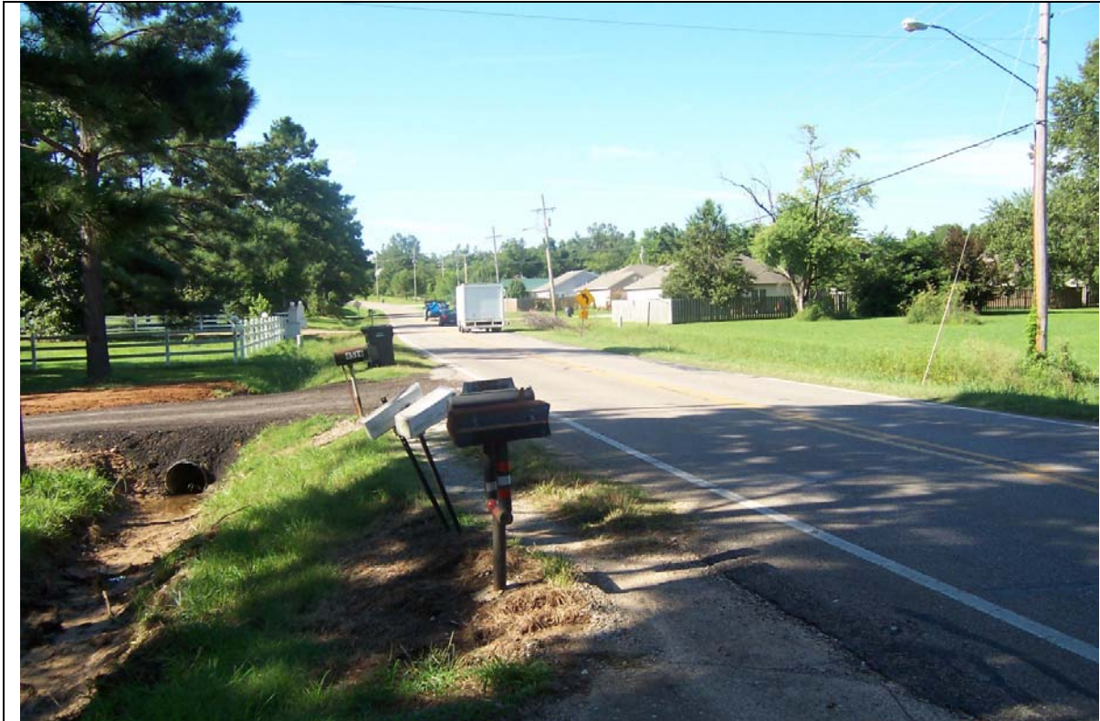
View looking south
