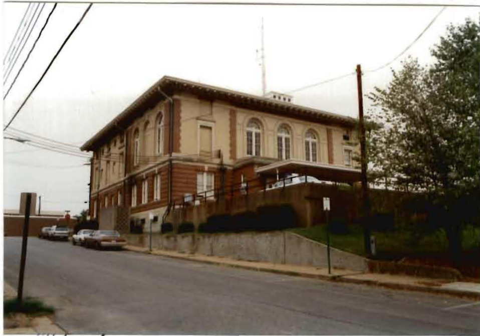
VIEW OF SUBJECT BUILDING FROM BACKSIDE, FROM JACKSON AVENUE
