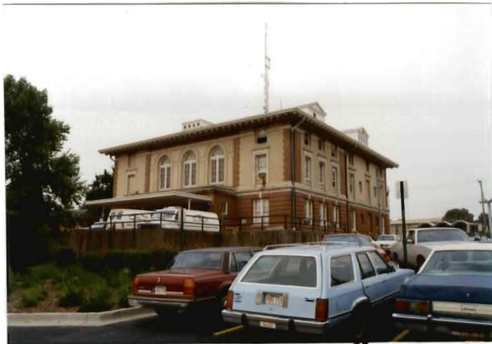
VIEW OF SUBJECT BUILDING FROM BACKSIDE, FROM ST. BERNARD'S PARKING LOT
