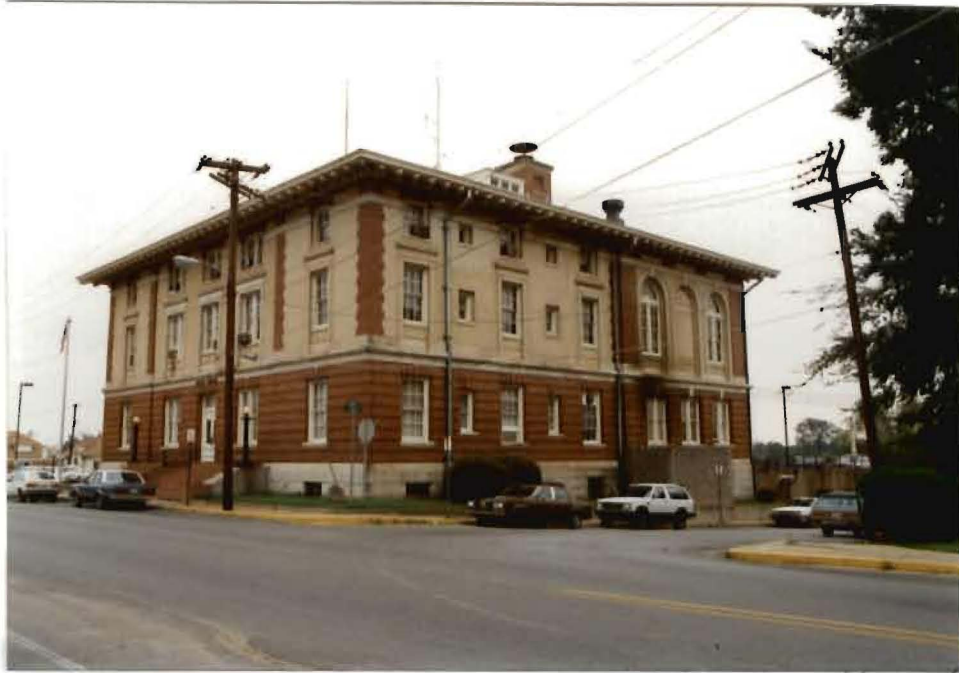
FRONT VIEW OF SUBJECT BUILDING WITH JACKSON AVENUE ON RIGHT AND CHURCH STREET ON LEFT
