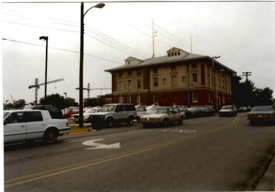
VIEW OF NORTH PARKING LOT AND SUBJECT BUILDING IN BACKGROUND
