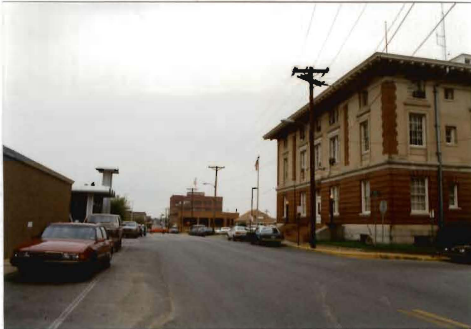
LOOKING NORTH ALONG CHURCH STREET, SUBJECT BUILDING ON RIGHT
