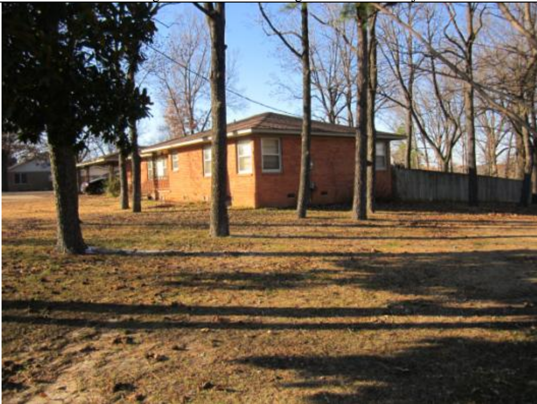
View looking northwest toward 2900 Stallings Lane located west of site.
